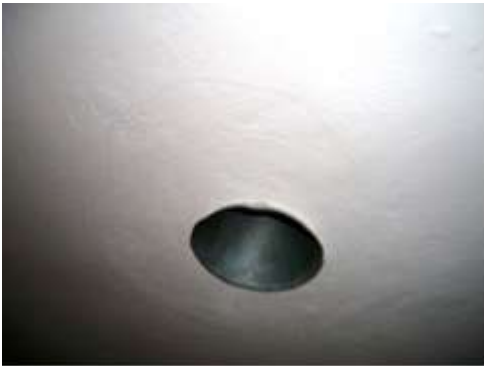
Photo 7: Rework to ceiling around shower head.
